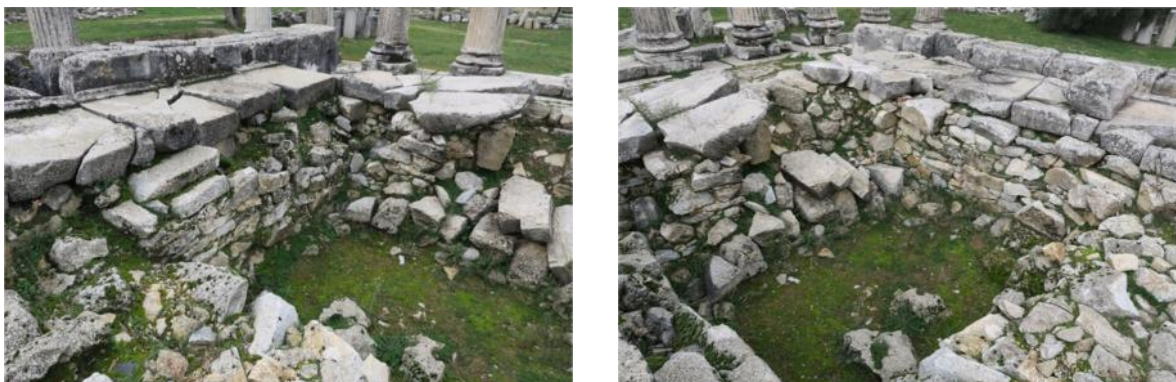
Figure 10-11: The wall of under the paving naos blocks
