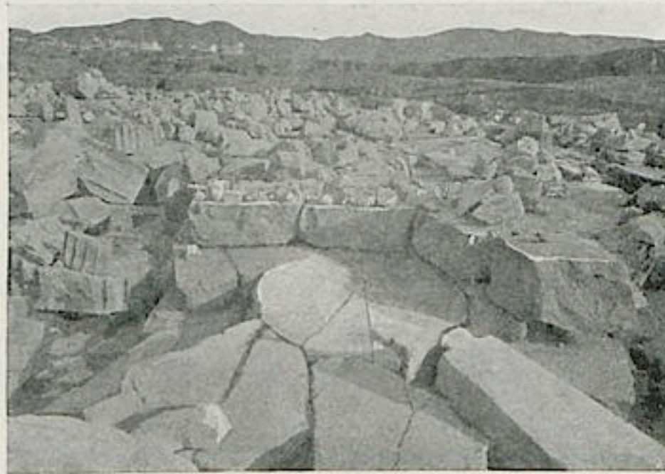
Fig. 70. D Column Plinth, chipped, and surrounded by E foundations.
