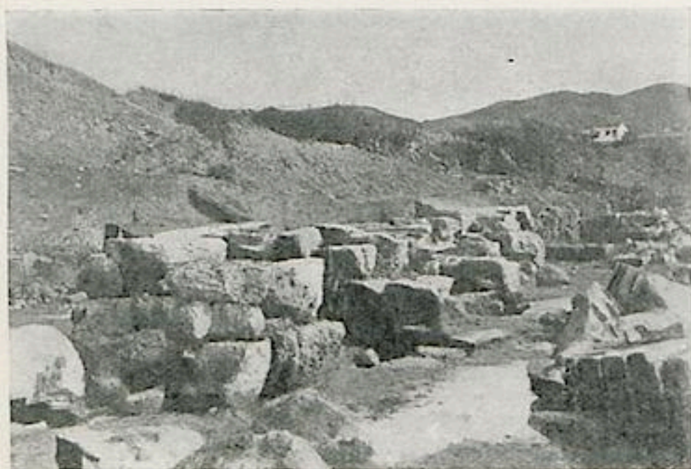
Fig. 6. Piers supporting Hellenistic Extension of Platform on the north side.
