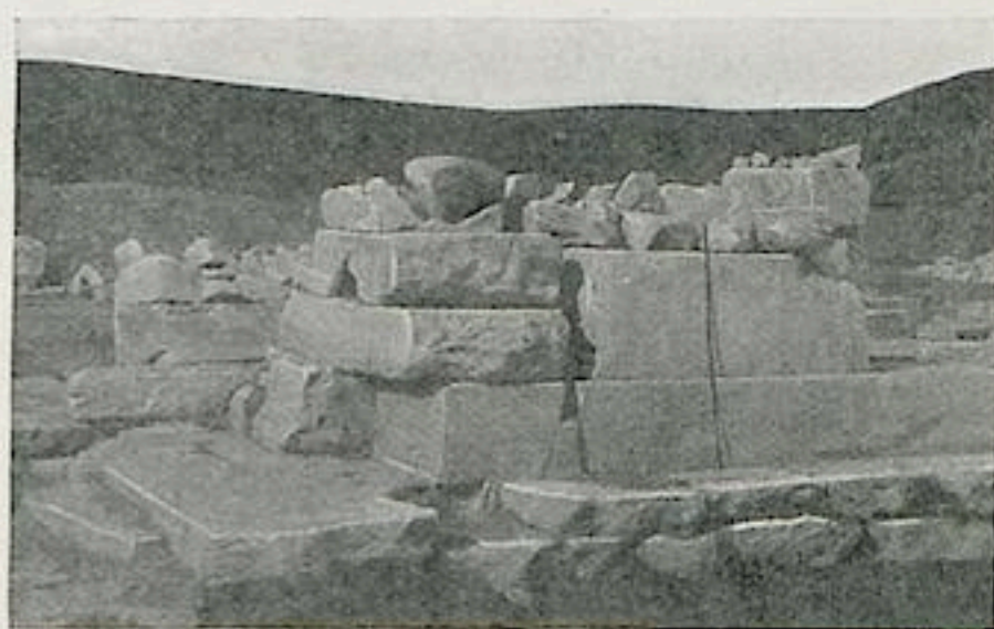
Fig. 68. Northern fragment of west wall of D cella , showing reveal of doorway.
