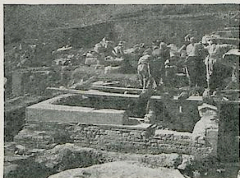
Fig. 17. N. Face of Basis, showing B walling under D coigns. A fragment of C enlargement seen projecting at the left (N.E.) corner.
