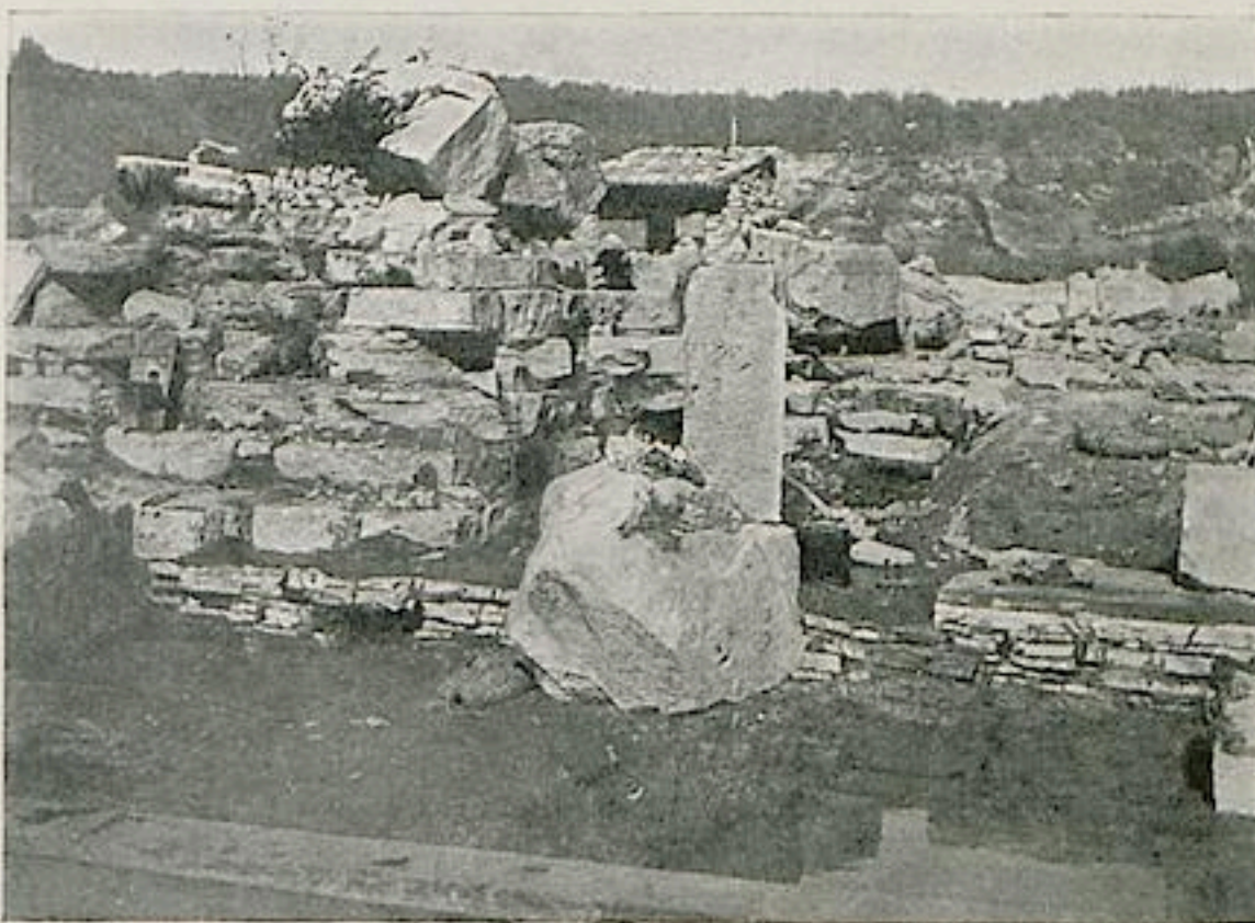
Fig. 23. C Western Enclosure Wall, seen under later foundation.
