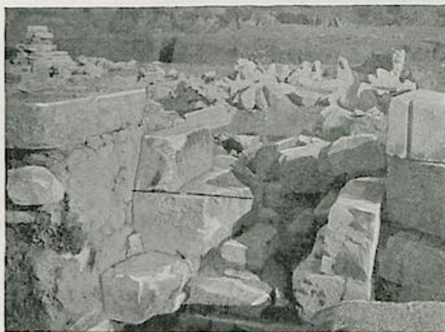
Fig. 66. S. wall of D cella , seen end on from the E. Facing courses on either side, and space for core between. Byzantine concrete on left in foreground.
