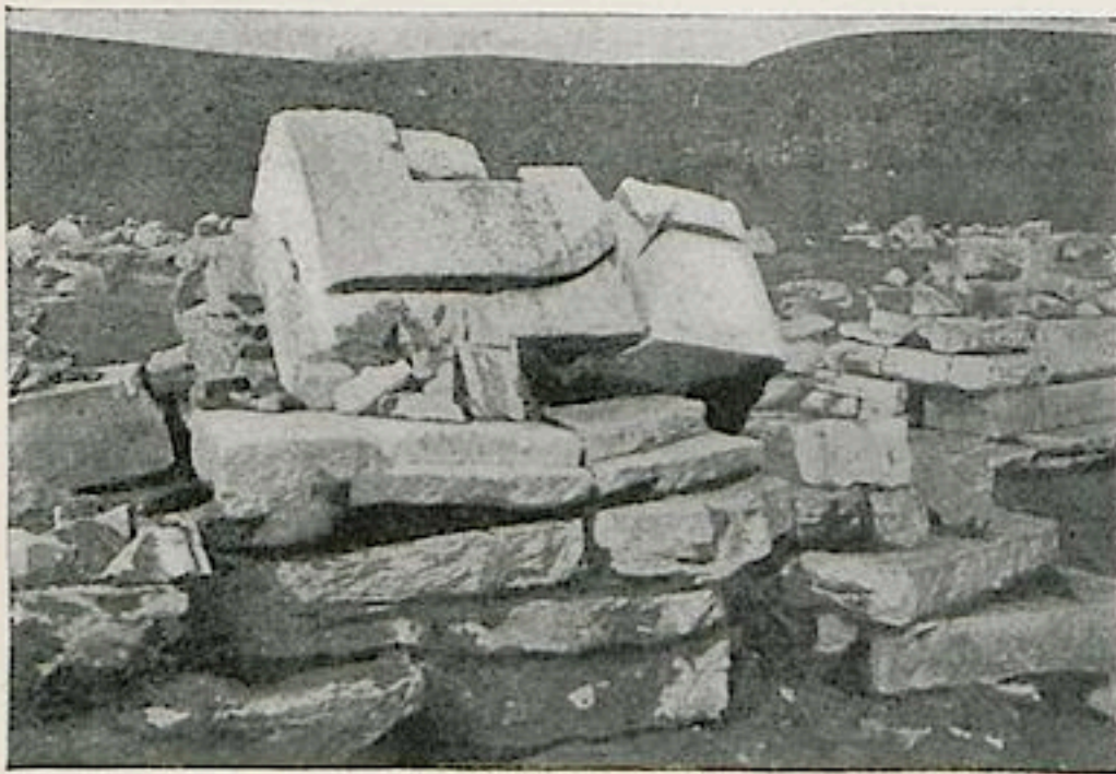
Fig. 1. Grooved Threshold Block, resting on Hellenistic foundations.
