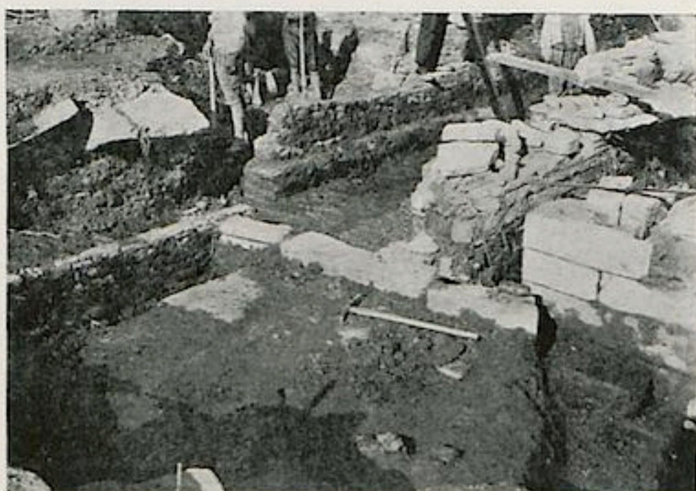
Fig. 22. Fragment of C (?) Foundation running along under W. wall of A Basis. B Thickening and Enclosing Walls seen behind.
