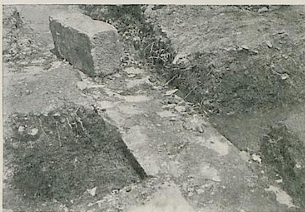
Fig. 26. Eastern Enclosure Wall of C . Lowest ashlar course preserved.
