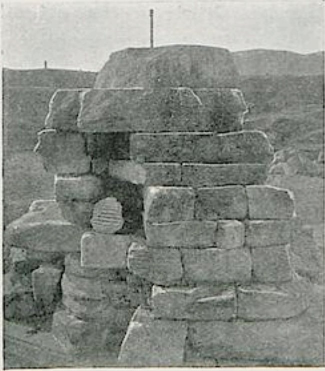
Fig. 69. N.E. column-base. D plinth seen built over with E foundations at left lower corner.
