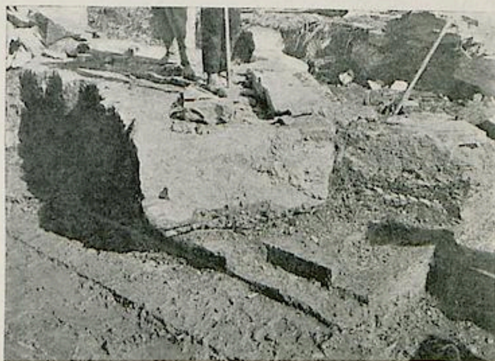
Fig. 12. Croesus Foundation Block bedded on B and C structures, in north part of D cella.
