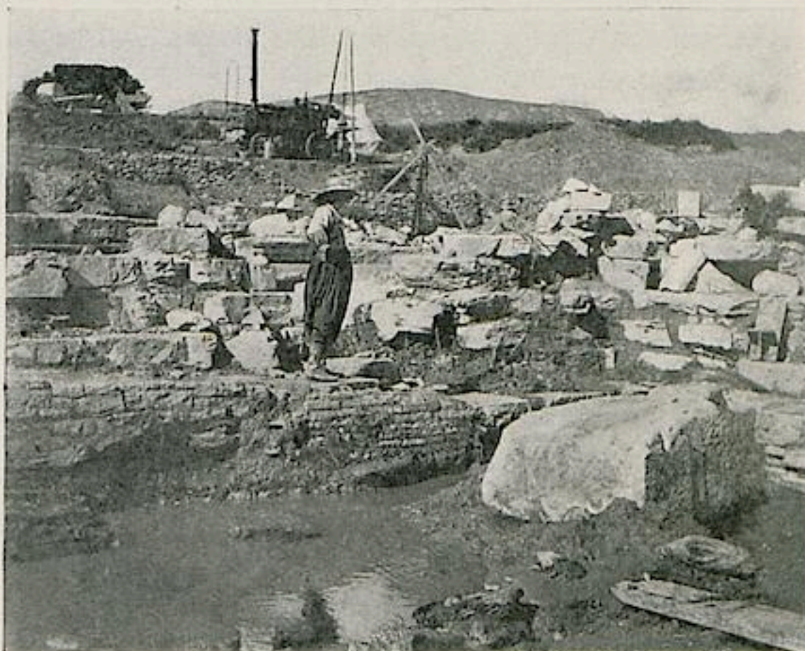
Fig. 28. Fragment of C Inner Enclosure on S.W. (under the man's feet). D Foundations continuing it on left, and foundations of D cella . S . Wall in background.
