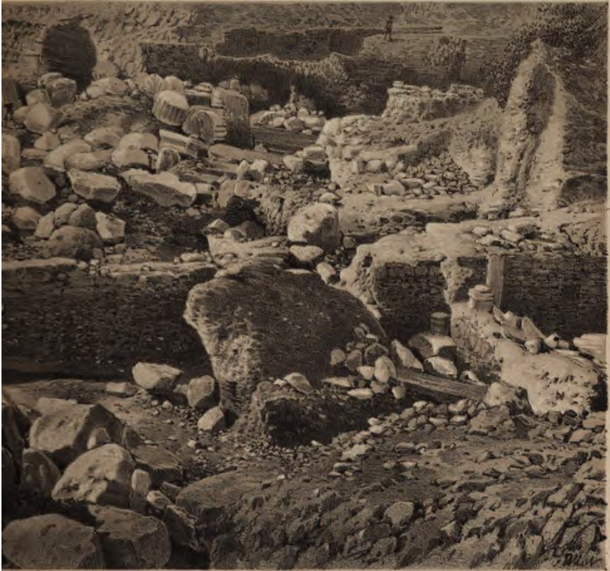
PLE, LOOKING WEST. DECEMBER 1871.
