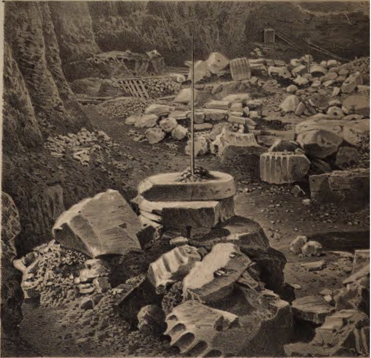
VIEW OF EXCAVATION ON SITE O
