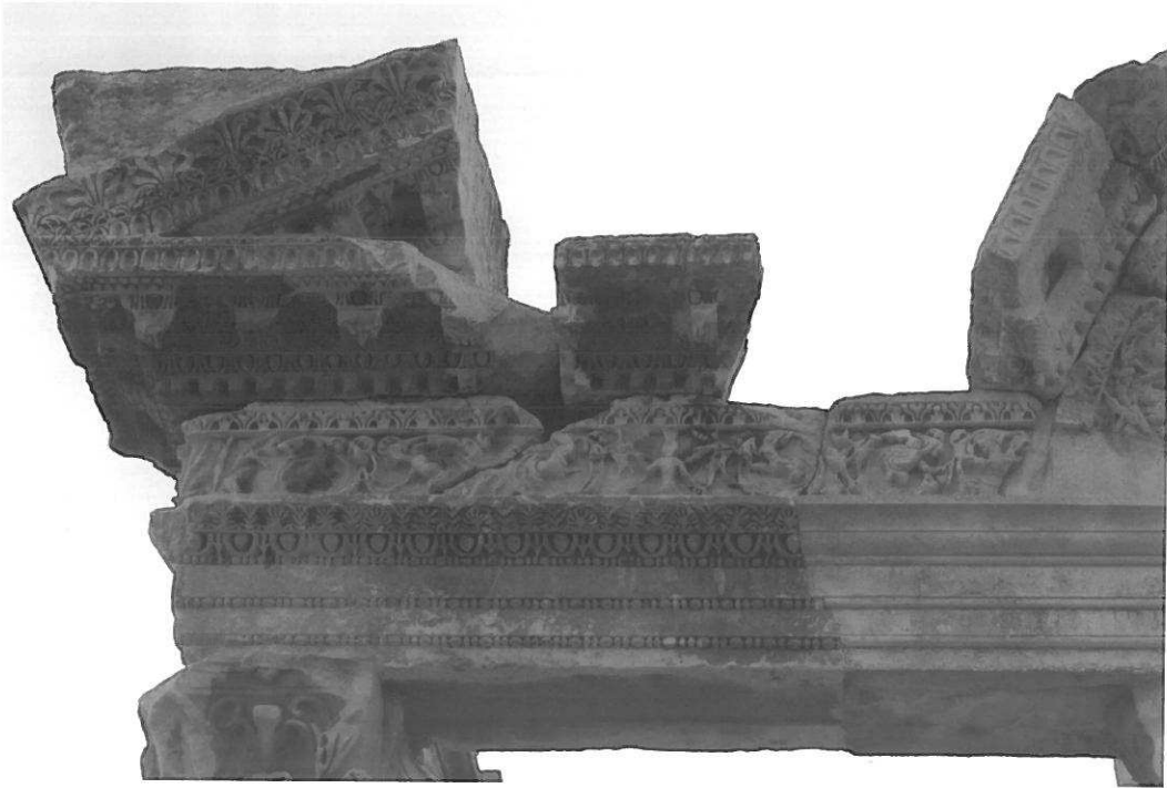
Fig. 10. Western horizontal architrave of the street façade, ancient replacement (© ÖAI).
