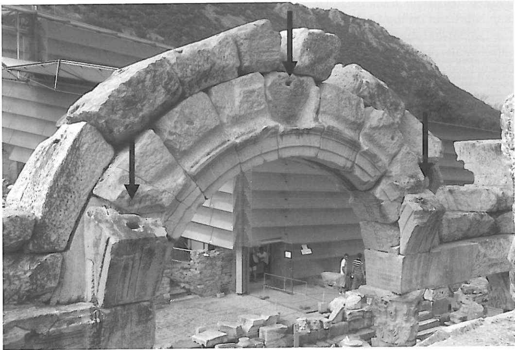
Fig. 16. Springings of three transverse arches at the back of the Syrian arcuated pediment (© ÖAI).
