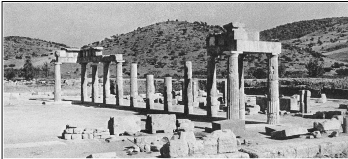
4. The stoa of Brauron as restored.
