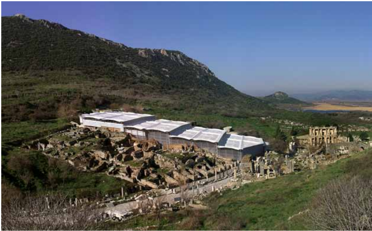
Terrace Slope House 2 protective roof in 2015 (Austrian Archaeological Institute, Niki Gail)
