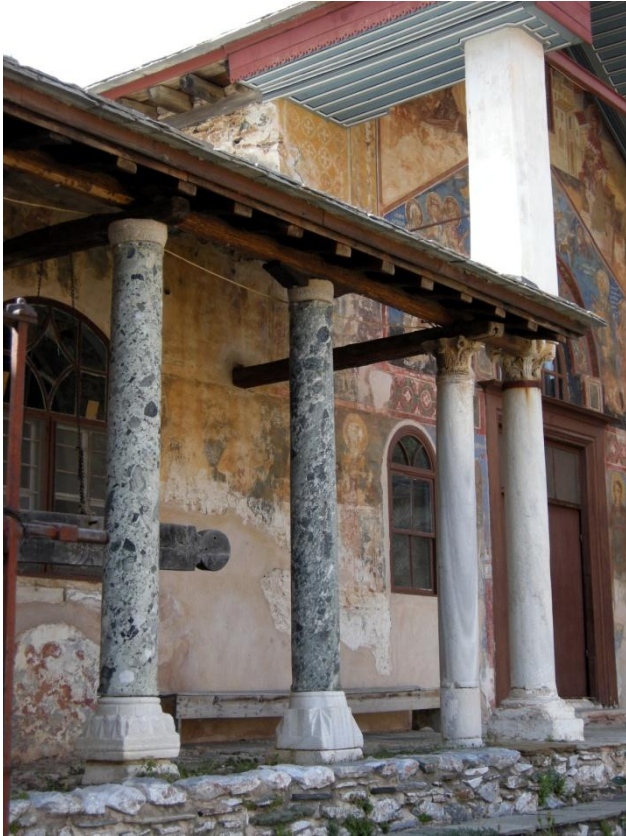
Figure 15: Capitals turned upside down at the bottom of the columns that support the porch below the Salutation.
