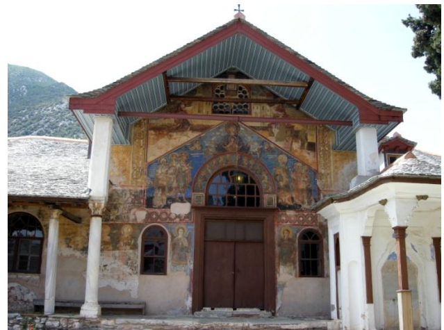
Figure 4: The facade of the refectory of the Great Lavra monastery.
