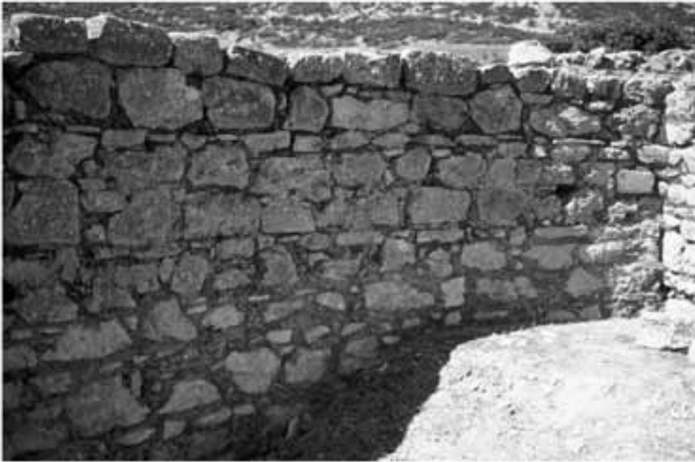
Taf. 20, 1: Raum A, Rundmauer – Innenschale
